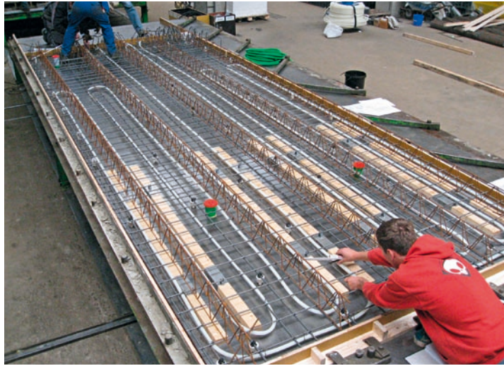
Displacement bodies and TBE ducts embedded at the factory in the precast bottom sandwich layer of a Ceiltec A floor
