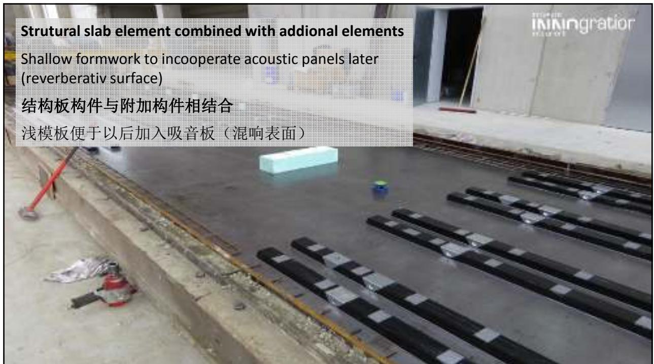
Precast slab element with different installation devices for multifunctional use
