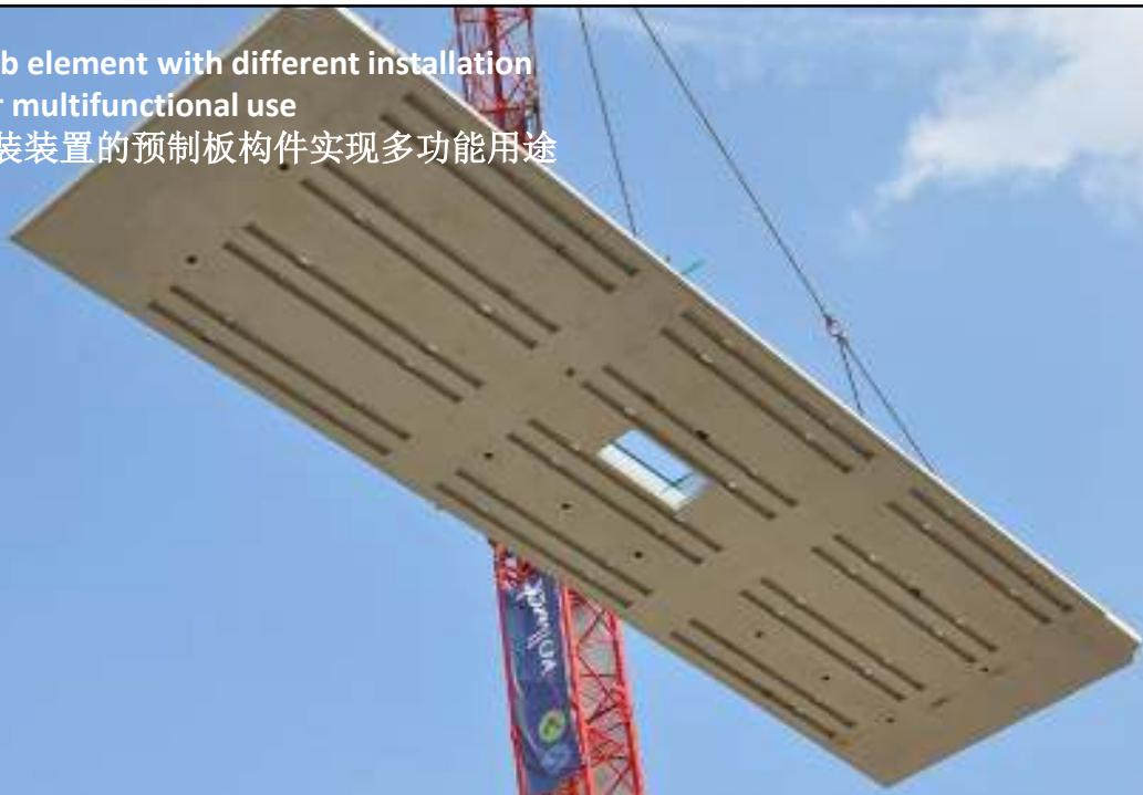
Precast slab elements with integrated building service elements
