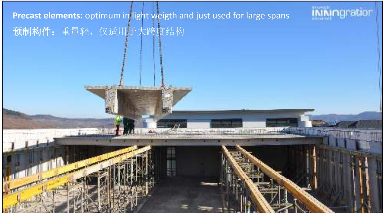
Precast elements: structural elements with prestressing
